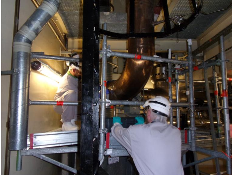
Typical conditions of UT inspections (EDF)
